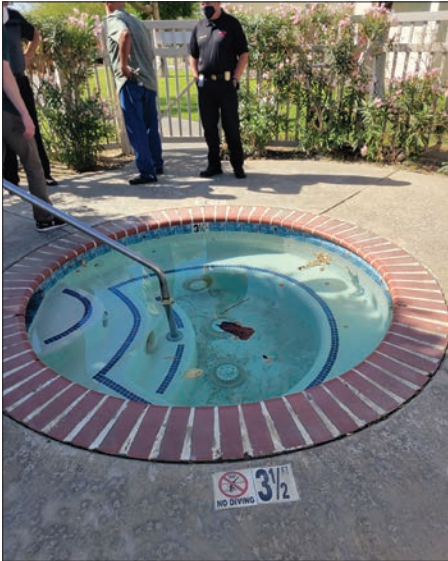
Photo 1. Staff from the Centers for Disease Control and Prevention (CDC) visually inspect a hot tub during a Legionella outbreak investigation. Legionella can grow and multiply in hot tubs that are not disinfected, cleaned, and properly maintained. Photo courtesy of Nakia Clemmons, CDC.
